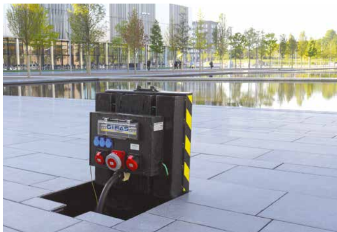
RETRANT 340x240x420mm Classification A15/ 15kN (1,5t)
