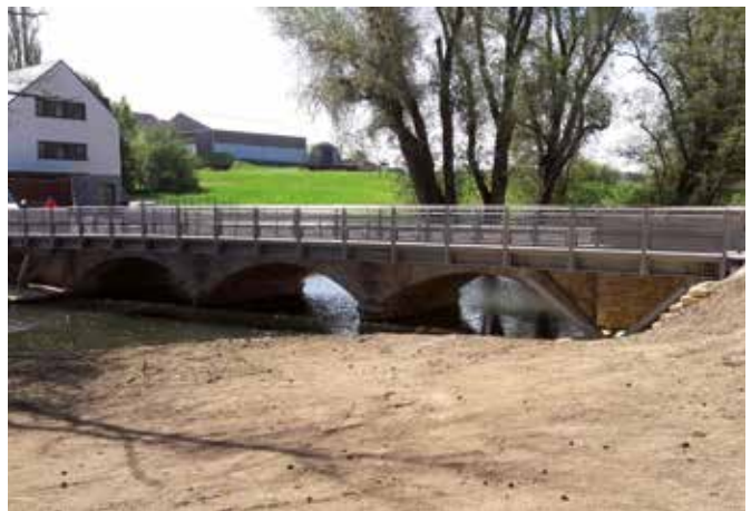
Pedestrian bridge, Wecker
