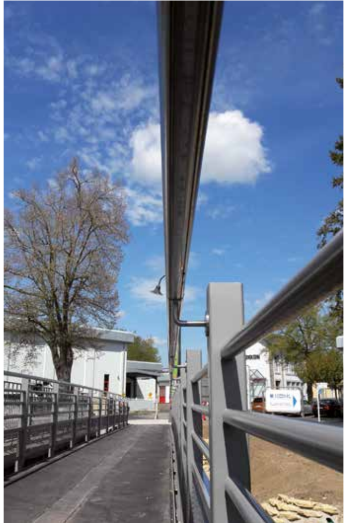
Pedestrian bridge, Wecker
