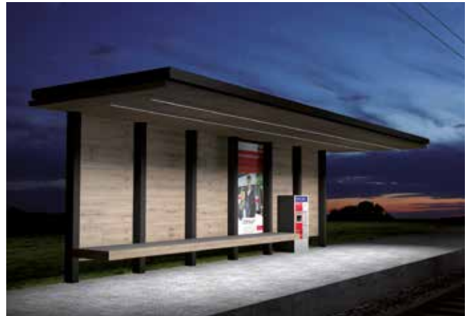
Station handling and waiting area
