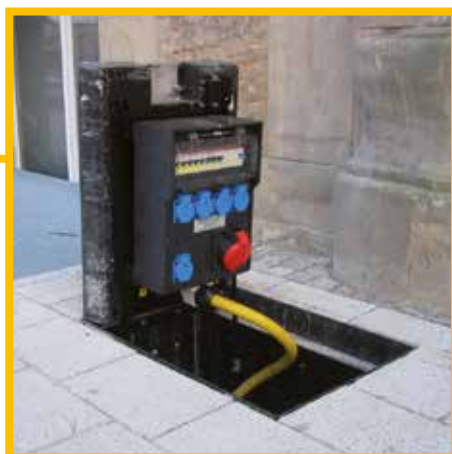
Fully installed CAMPETTO
