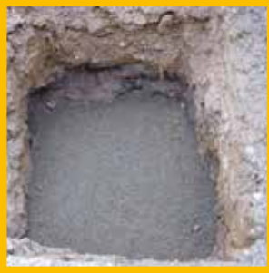
Excavating the installation pit
