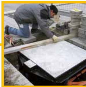
Levelling of the whole unit
