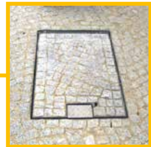
Adaptation to the surroundings with filler material
