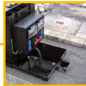
Decanting and concreting-in
