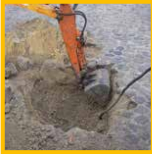
Excavating the installation pit
