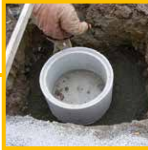
Customer-side concrete ring
