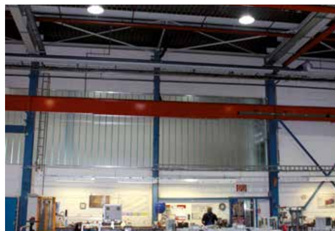
High bay lighting
