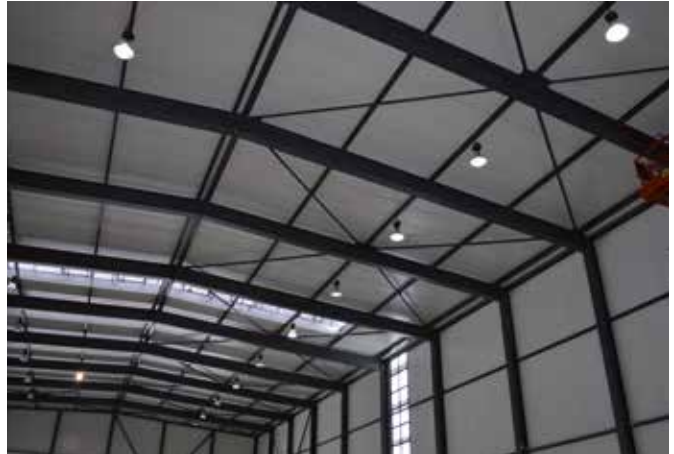
High bay lighting
