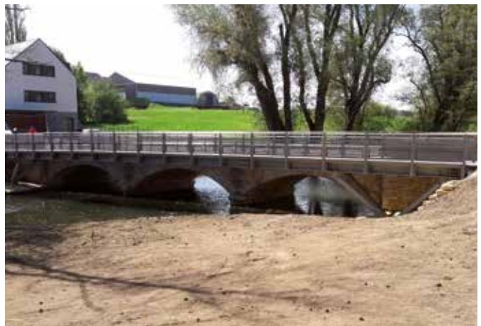
Pedestrian bridge, Wecker
