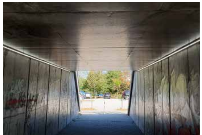
Lighting underpass, Oberkirch
