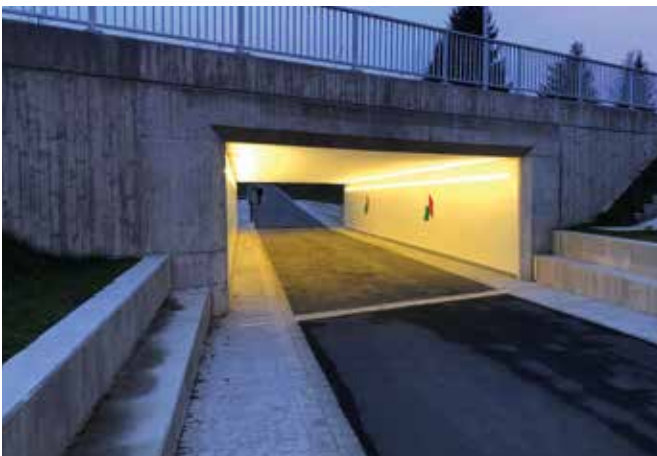
Lighting underpass, Weiden
