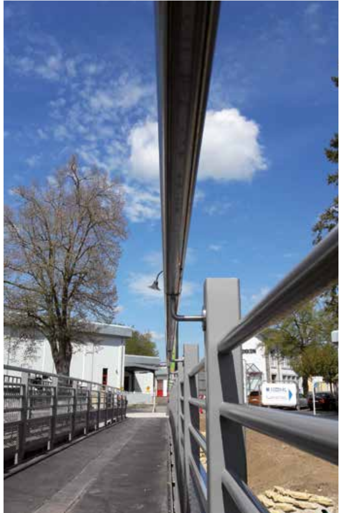
Pedestrian bridge, Wecker
