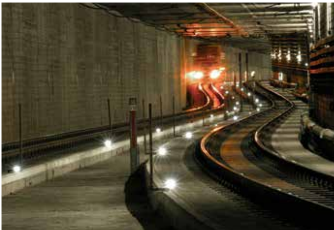
U-Bahn Tunnel, MarkLED
