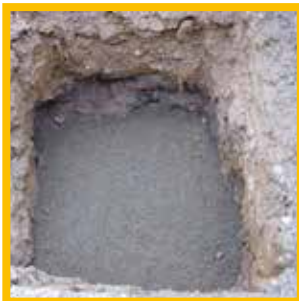
Excavating the installation pit
