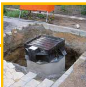
Insertion of the entire unit into the prepared installation pit
