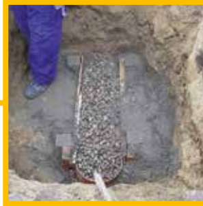
Topping up the installation pit
