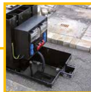
Decanting and concreting-in
