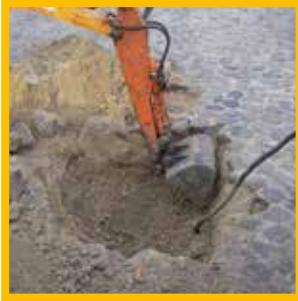
Excavating the installation pit
