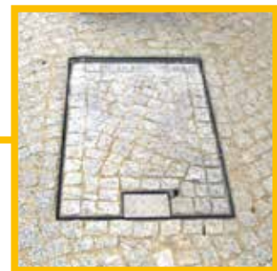
Adaptation to the surroundings with filler material
