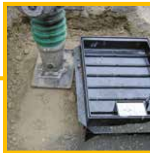
Decanting and concreting-in
