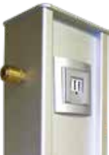
Compressed air and data socket
