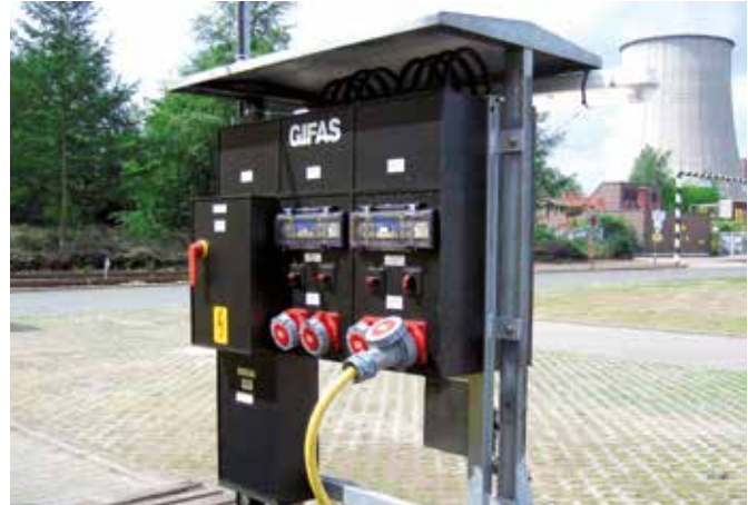
Wall mounted distributor
