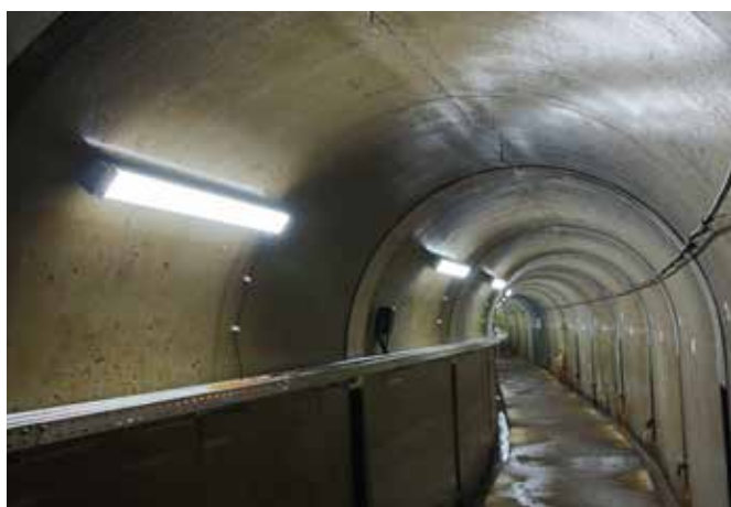
Inspection shaft lighting
