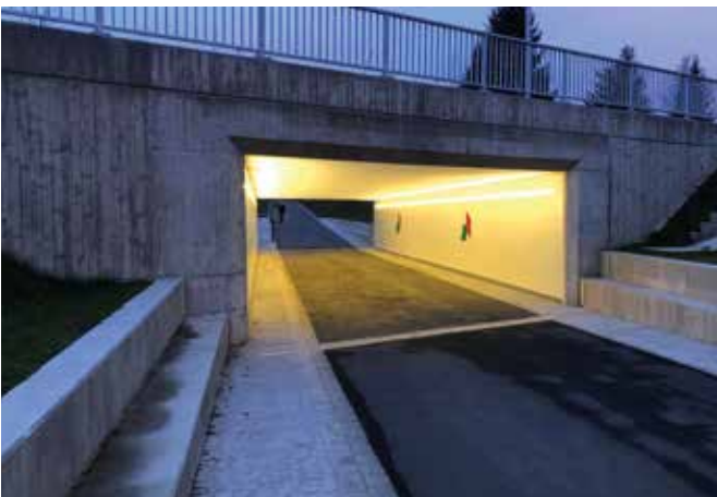
Lighting underpass, Weiden
