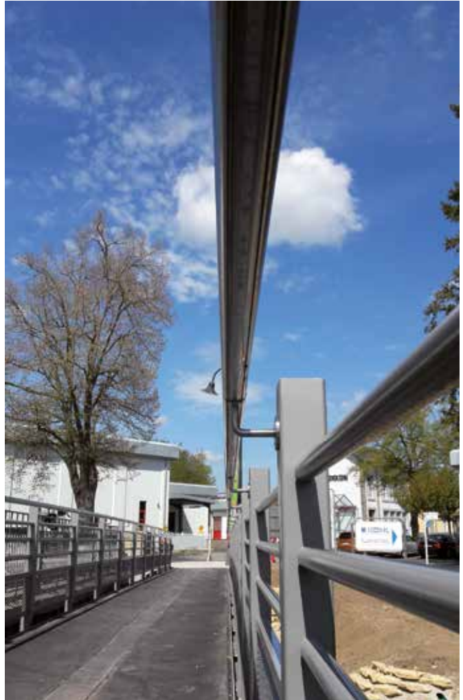
Pedestrian bridge, Wecker
