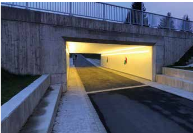
Lighting underpass, Weiden
