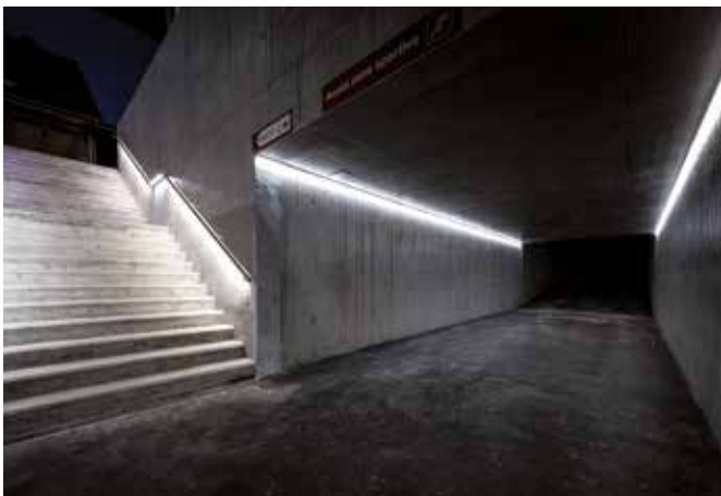
Railway station, Sembranch (Underpass: LaneLED WALL, Stairs: LaneLED INOX42)
