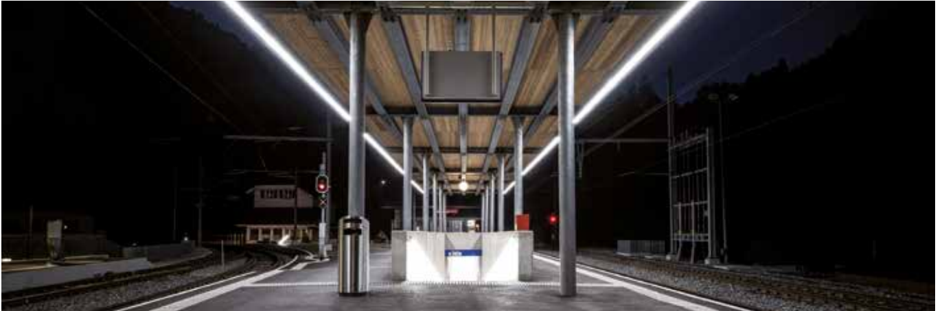
Railway station, Sembranch (Underpass: LaneLED WALL, Stairs: LaneLED INOX42)
