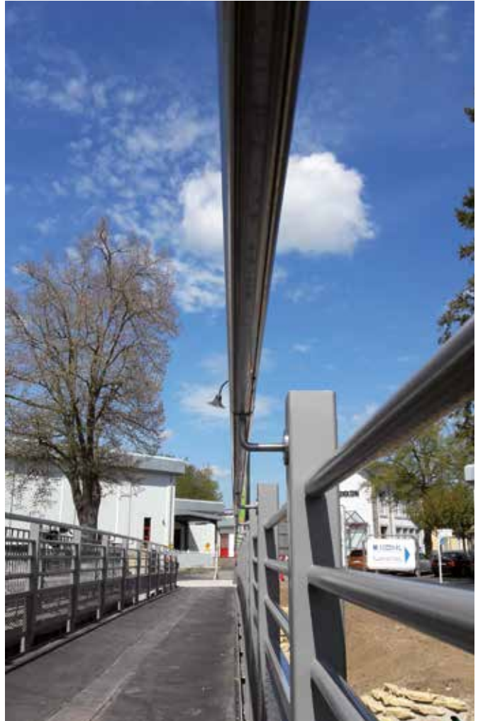
Pedestrian bridge, Wecker
