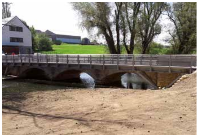
Pedestrian bridge, Wecker
