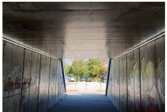
Lighting underpass, Oberkirch
