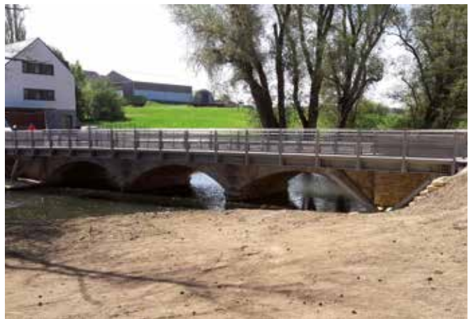
Pedestrian bridge, Wecker
