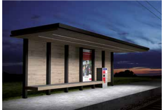
Station handling and waiting area
