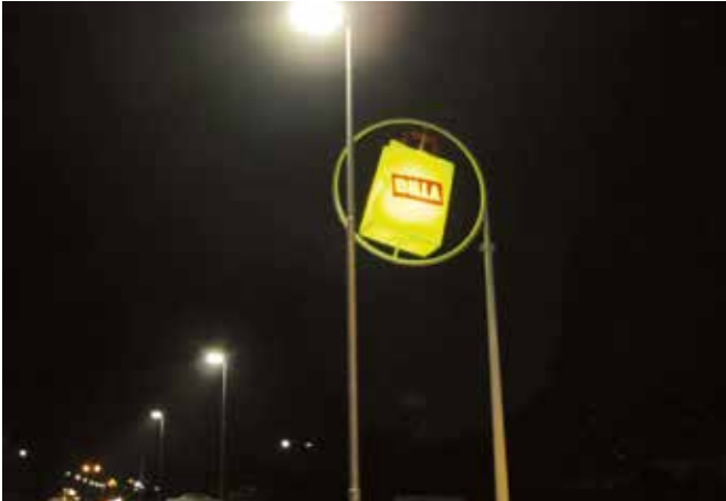
Car park lighting Billa, Mistelbach
