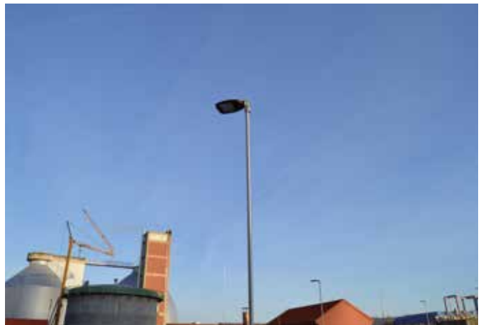
Sewage treatment plant, Osnabrück
